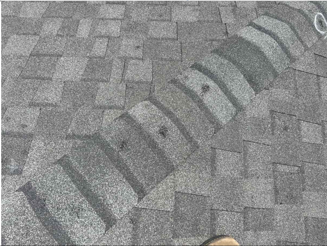
Left Slope Hail Damage
