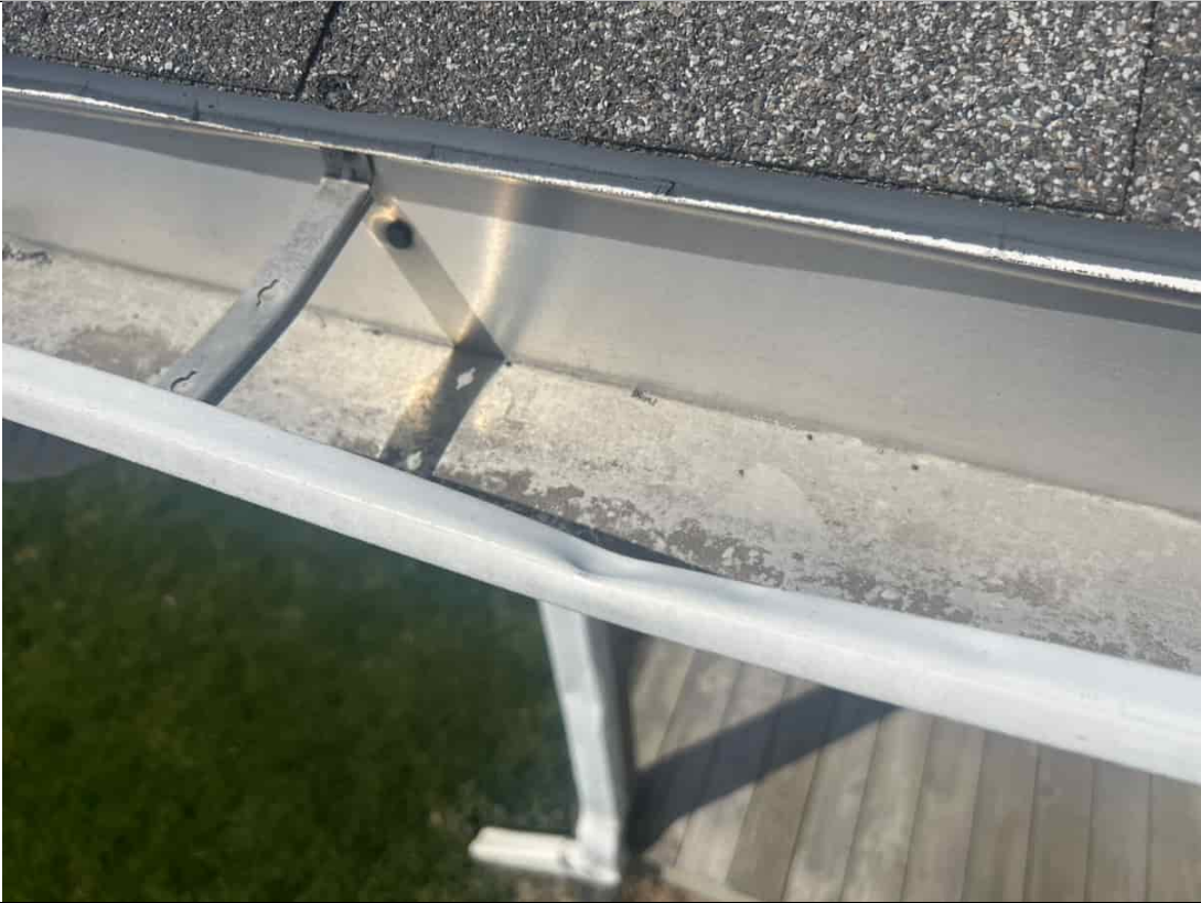
Gutter Damage
