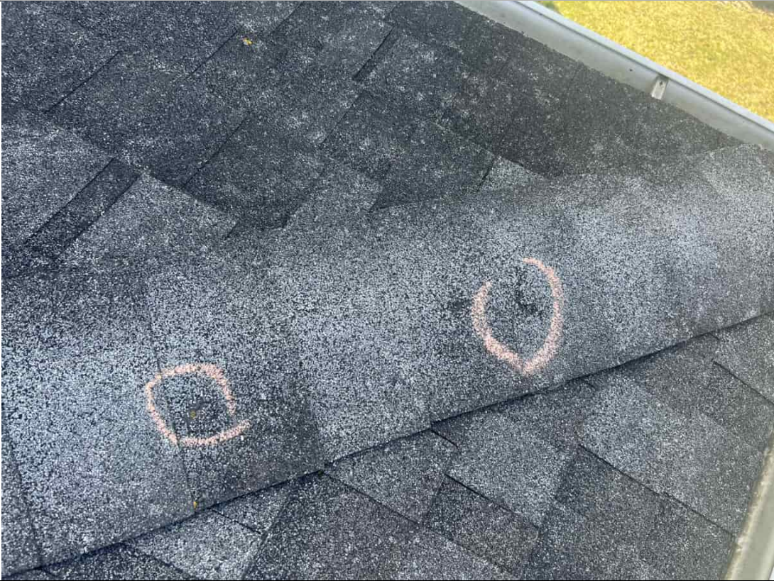
Right Slope Hail Damage
