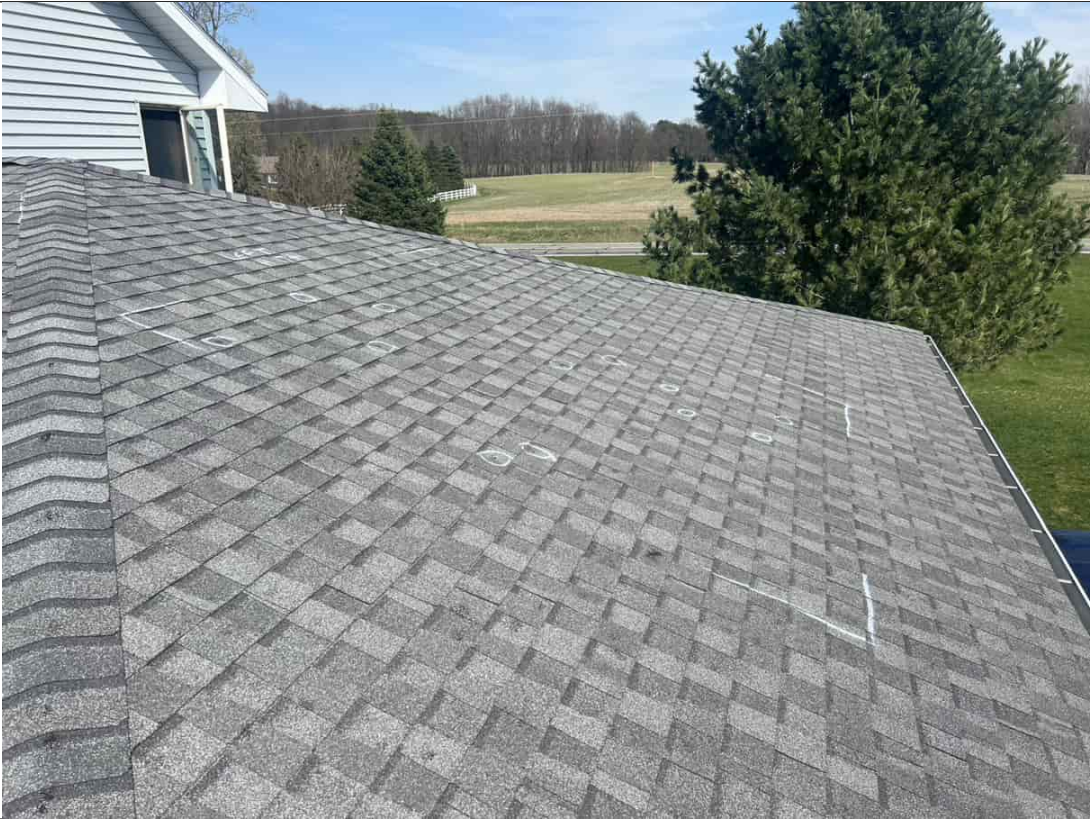
Left Slope Hail Test Square
