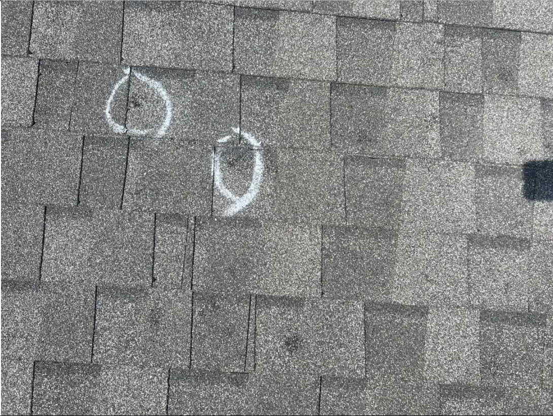
Back Slope Hail Damage
