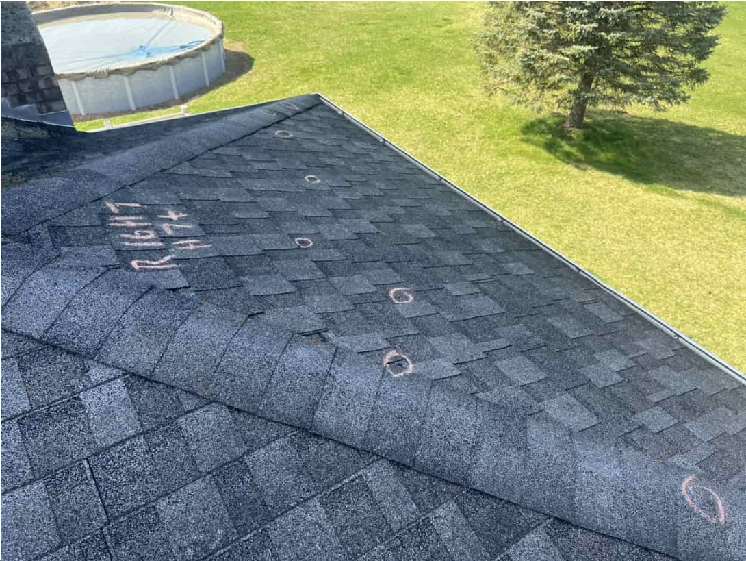
Right Slope Hail Damage
