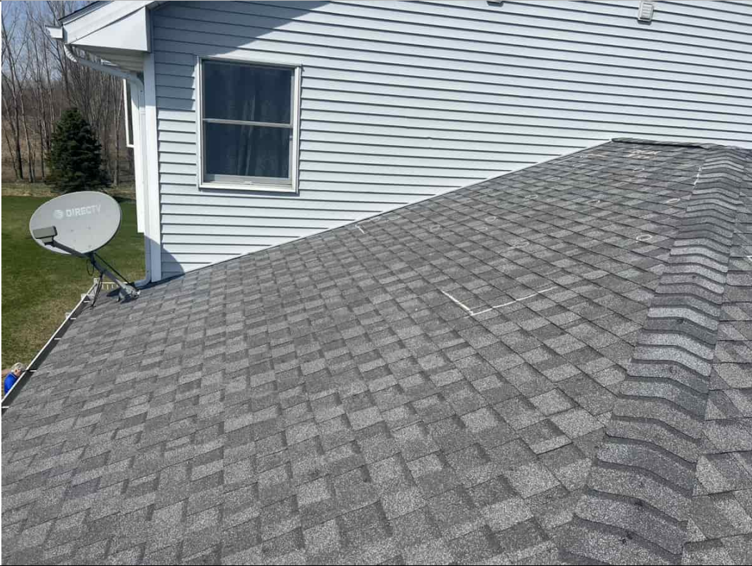
Back Slope Hail Test Square
