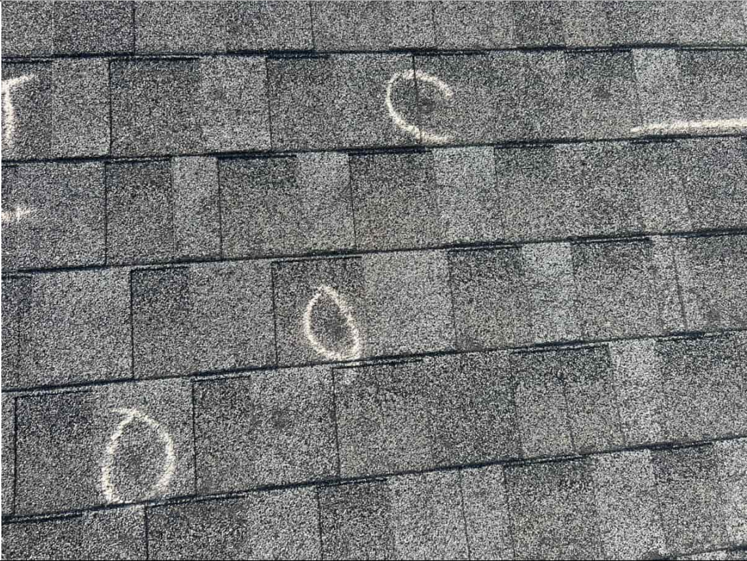
Front Slope Hail Damage
