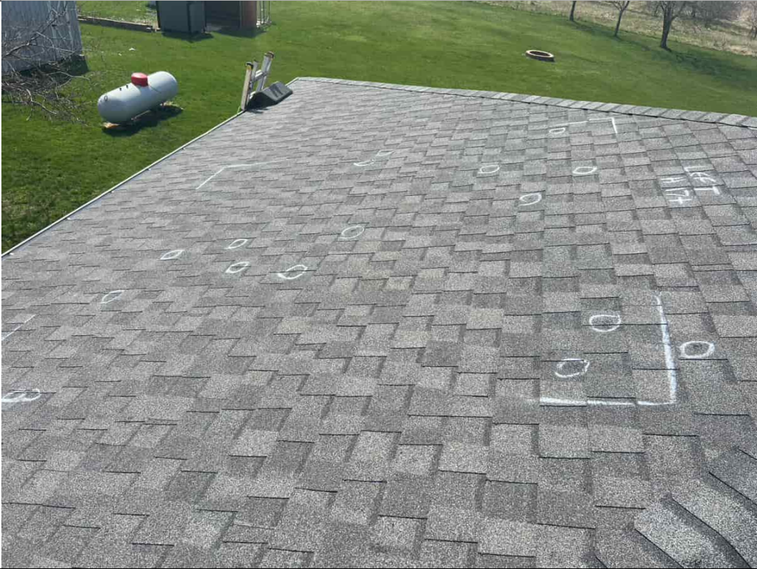
Left Slope Hail Test Square
